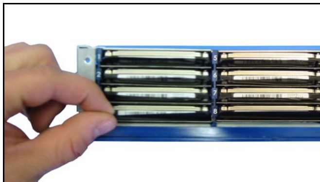
Figure 3-20 Pulling out the failed disk drive.
